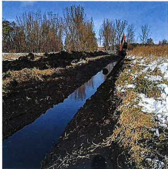
Typical ditch cleaning.
