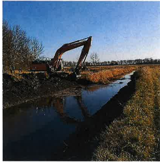
Typical open ditch cleaning.
