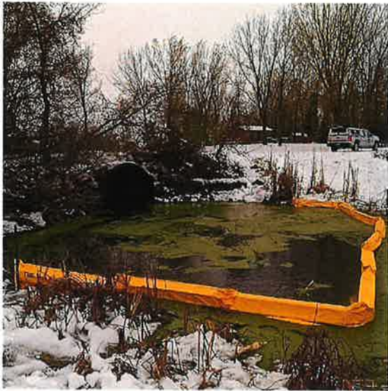
Floatation silt fence installation.
