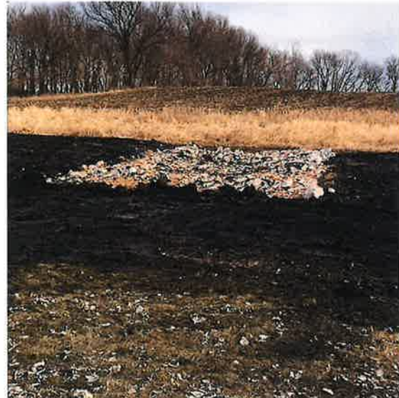
Typical spillway overflow rip rap area.
