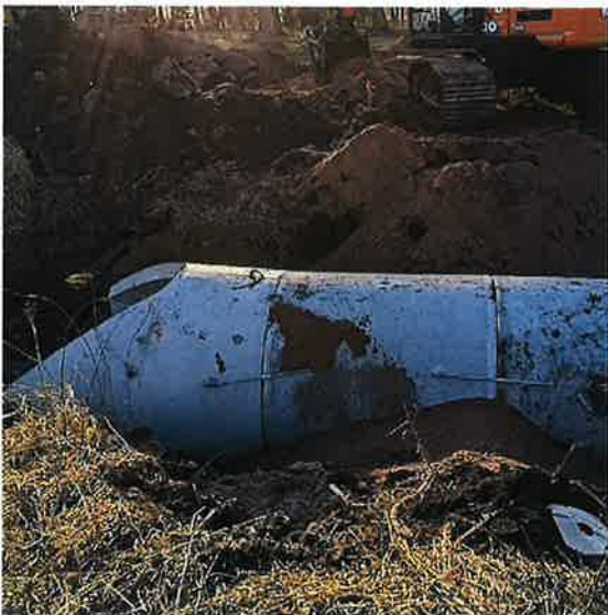
Road crossing at station 0+00.
