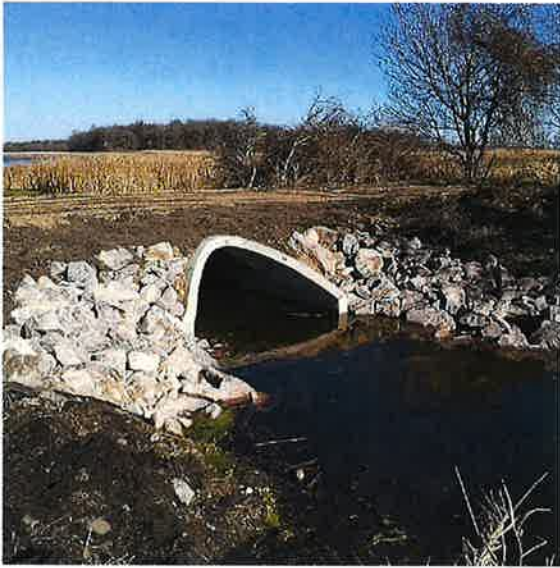
Finished road crossing at station 0+00 South.
