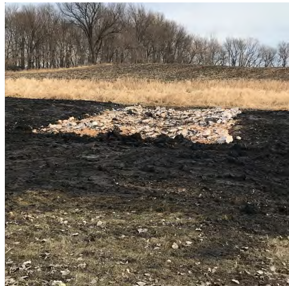
Typical spillway overflow rip rap area.
