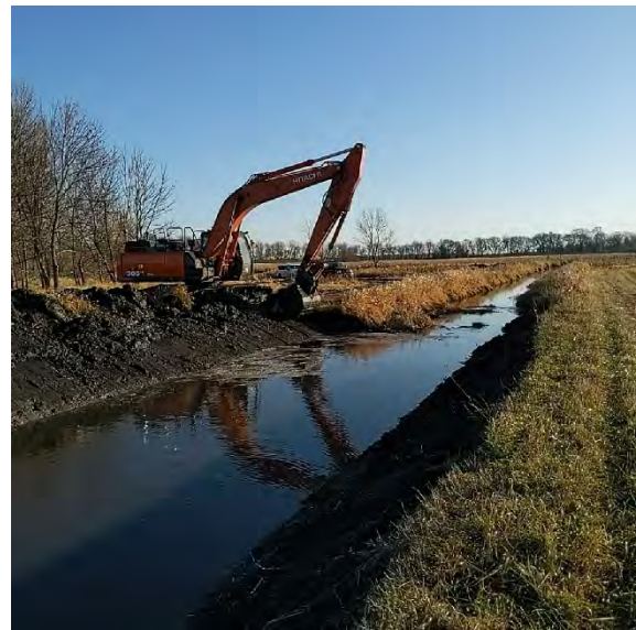
Typical open ditch cleaning.
