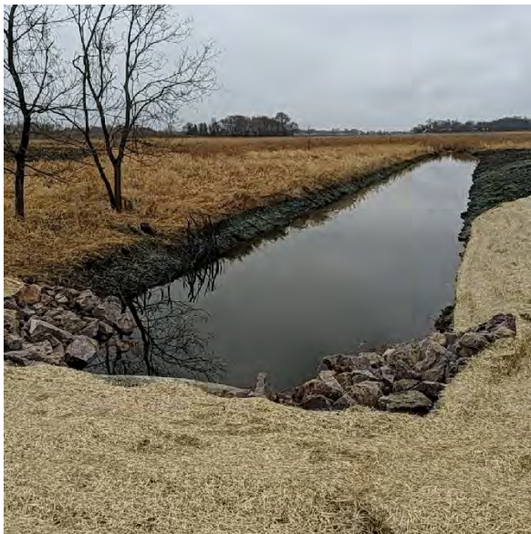
Typical seeding and blanketing procedure.
