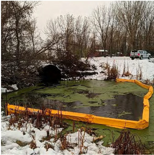
Floatation silt fence installation.
