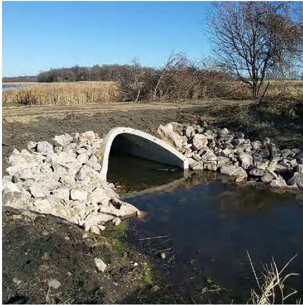
Finished road crossing at station 0+00 South.
