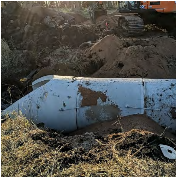
Road crossing at station 0+00.
