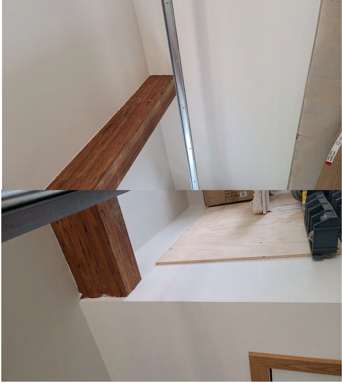
Another view of the LVL at the front (streetside) of the garage.
