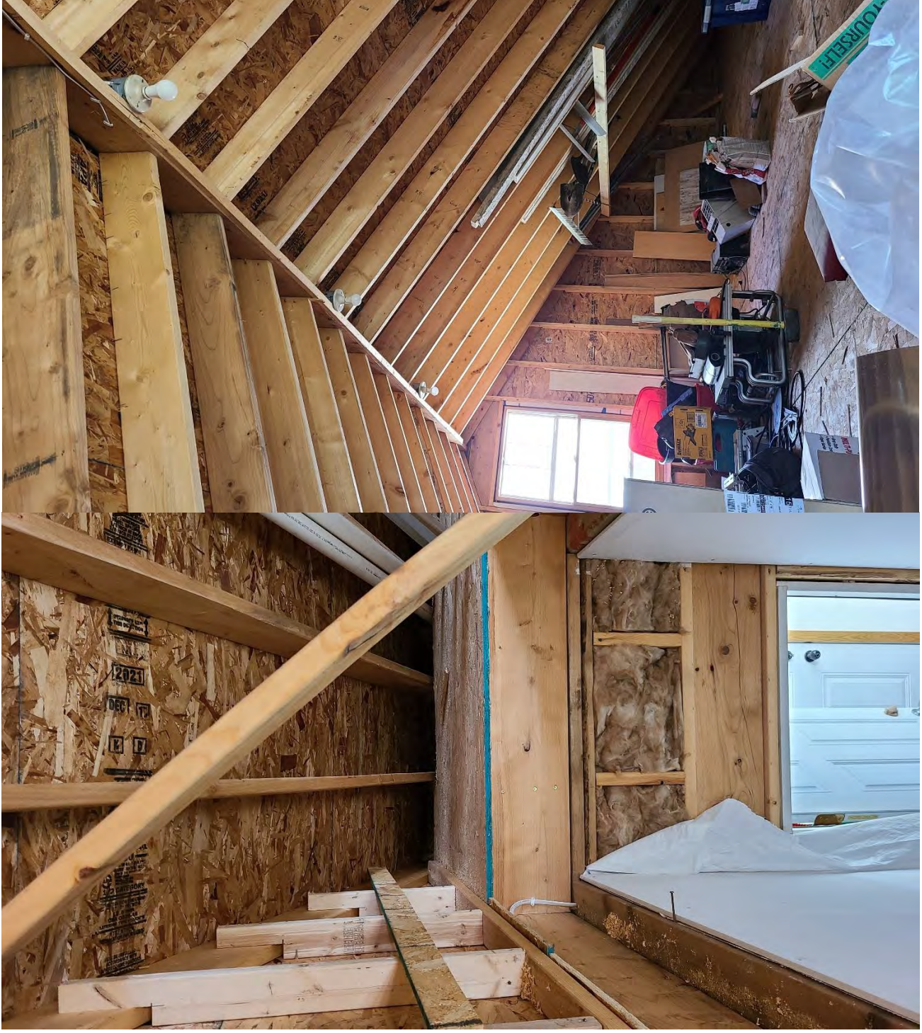
Left photo view of roof rafters resting on the front LVL beam. Right photo a view of the attic storage space.
