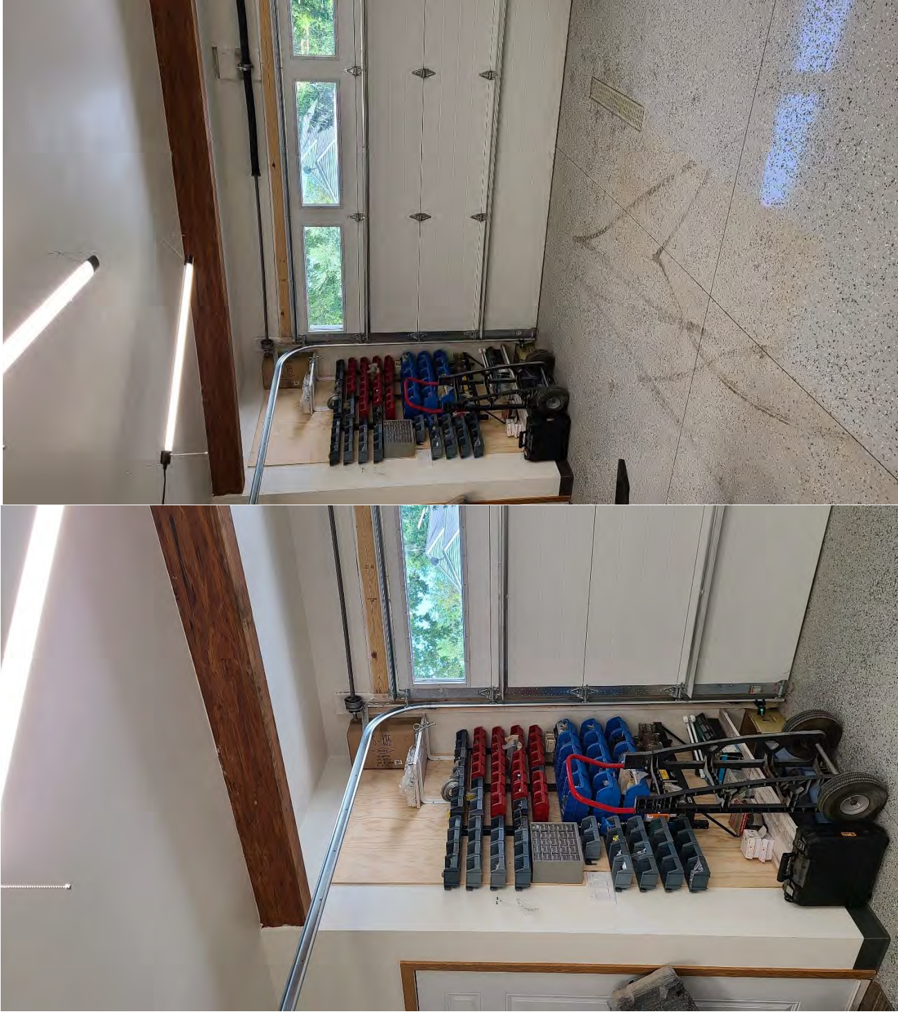
Left and Right Photos. View of design and LVL beam across the front (street side) of the garage.
